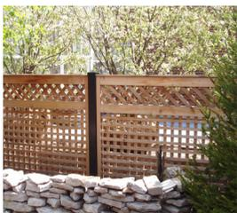
Another alternative is to substitute pressure treated lumber. Pressure treated fence posts will last up to thirty years without rotting, and pressure treated fences are generally less expensive than cedar. But there are some drawbacks to this material for use in fences:
